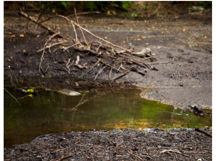
On Tuesday the extent of sediment build-up in Carter Pond is evident. In addition to sediment, trees and logs must be removed.
