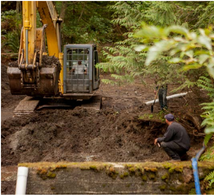
Jamie Weismiller, the J&E excavator operator, can move a lot of material with the 1 yard bucket.
