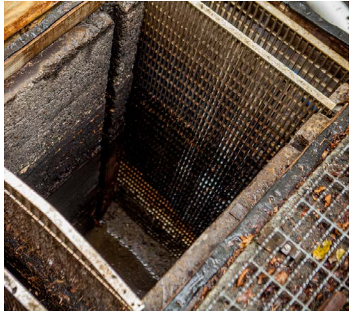
While the excavator removes sediment, BIFWC volunteers remove and clean the 8 heavy hatchery water intake filter grates. Note all the sediment build-up on the grates and that about 3 feet of mud and silt has accumulated at the bottom of the water intake structure right in front of the water intake pipe opening.
