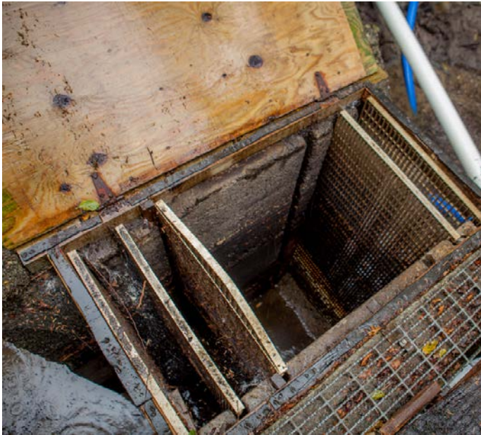
While the excavator removes sediment, BIFWC volunteers remove and clean the 8 heavy hatchery water intake filter grates. Note all the sediment build-up on the grates and that about 3 feet of mud and silt has accumulated at the bottom of the water intake structure right in front of the water intake pipe opening.
